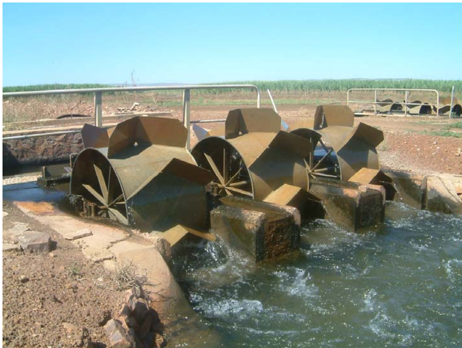
Detheridge wheels monitor the flow of water onto farms.
