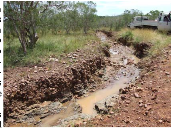
Figure 5: Gully from scoured out roadside V-drain.
